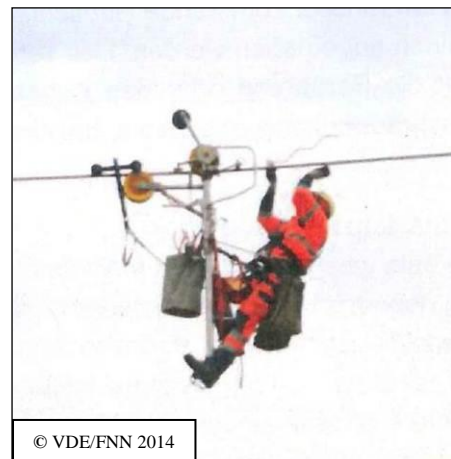
Figure 9-2: Installation of bird diverters using a line car (left) or a line bicycle (right)
