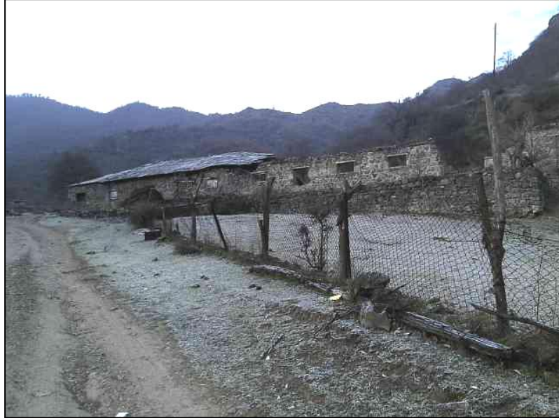
Photo 6-3: Farmhouse located in the planned line corridor
