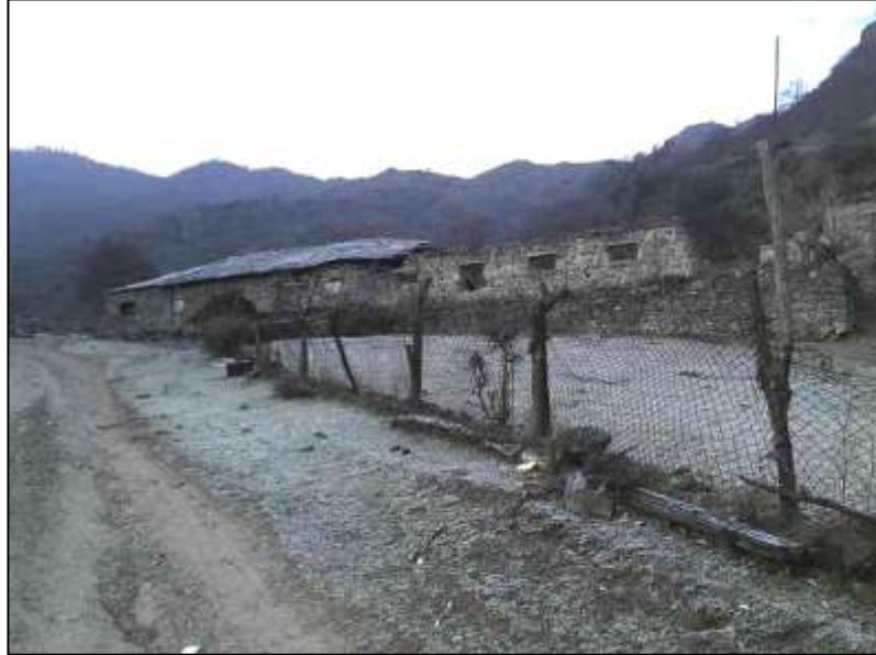
Photo 6-3: Farmhouse located in the planned line corridor
