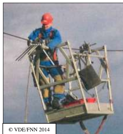
Figure 9-2: Installation of bird diverters using a line car (left) or a line bicycle (right)
